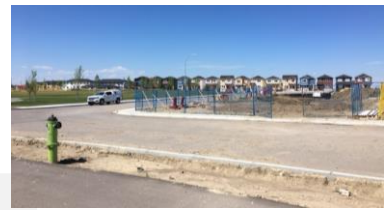
Current Belvedere residential construction (North of Site)
