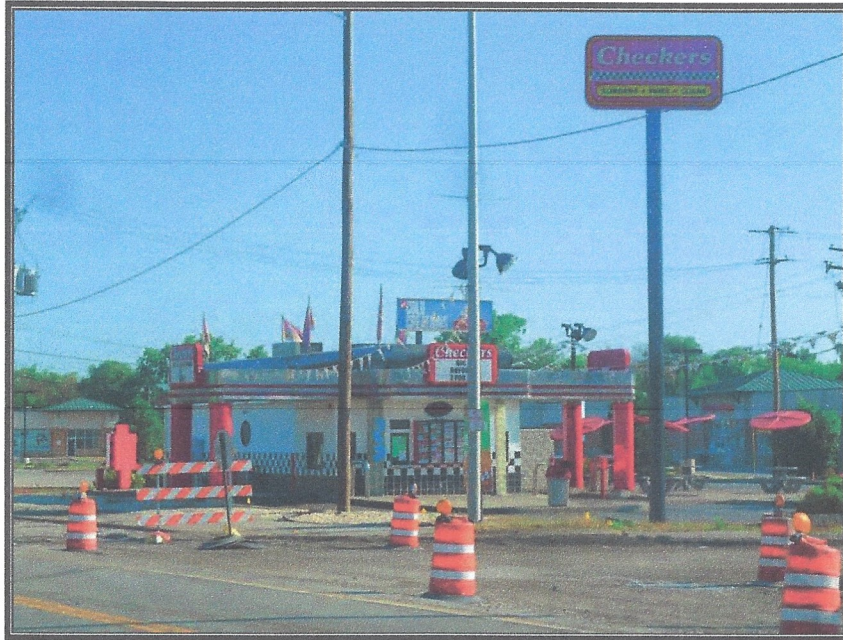
View of subject property from southwest
