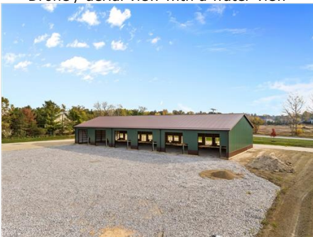
View of front facade
