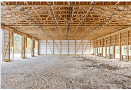
View of miscellaneous room
