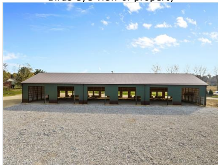
View of front facade with an outbuilding
