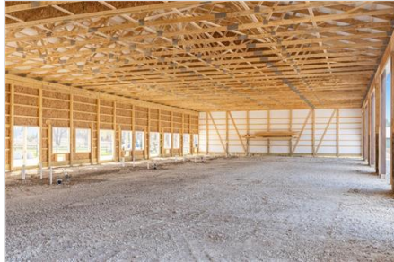
Misc room with a towering ceiling
