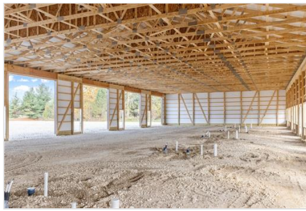
View of miscellaneous room
