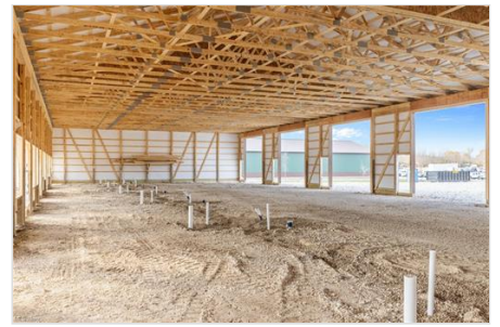
View of miscellaneous room
