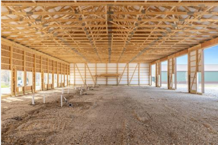
View of misc room
