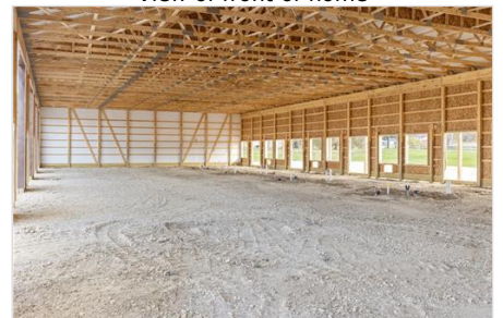
View of miscellaneous room
