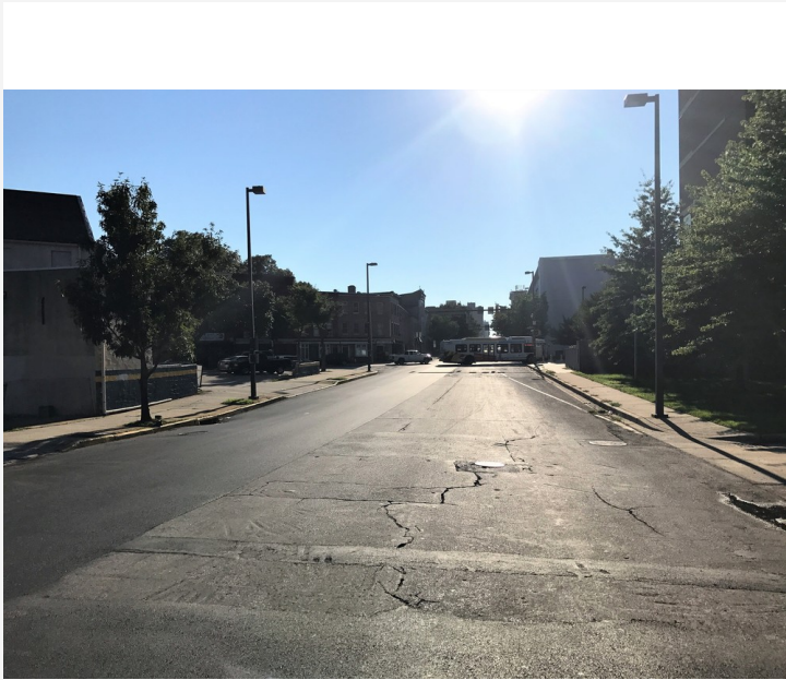
East View on Franklin Street
