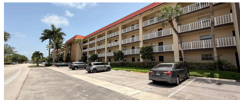
Building exterior & resident parking
