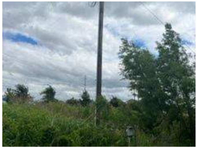
Photo #20 Far East / South Facing South Electrical Dropdown
