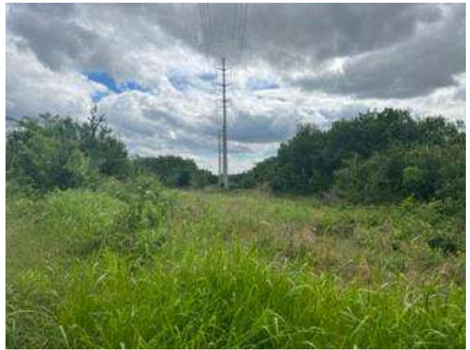
Photo #28 Mid East / North Facing North
