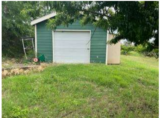
Photo #18 Far East / Metal Building North End
