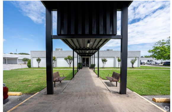
1600 - 1610 Connecting Canopied Walkway
