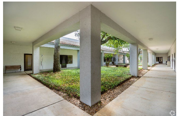
1600 Atrium Entrance Walk
