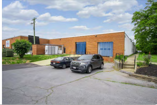
View of Dock Door
