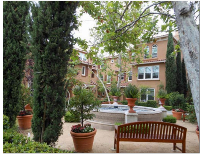
The side courts of these two buildings work together to create a single space.
