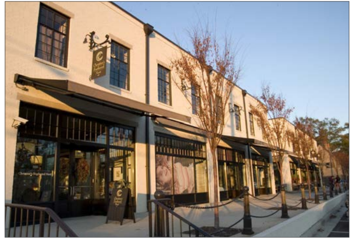
Shopfront Example - large glazing area of display windows, glass door, clerestory and retractable awnings.
