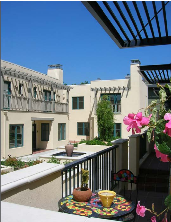
The side yard of this multi-family building provides access to adjoining units.
