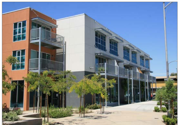
The orange mass of this mixed-use building is set back from the rest of the building. Further articulation is provided by second- and third-story balconies.
