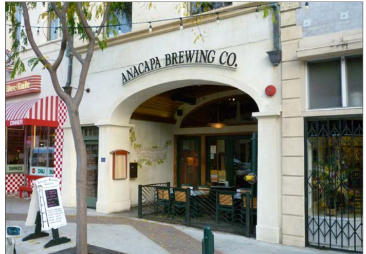
A recessed storefront accommodates covered, outdoor seating.
