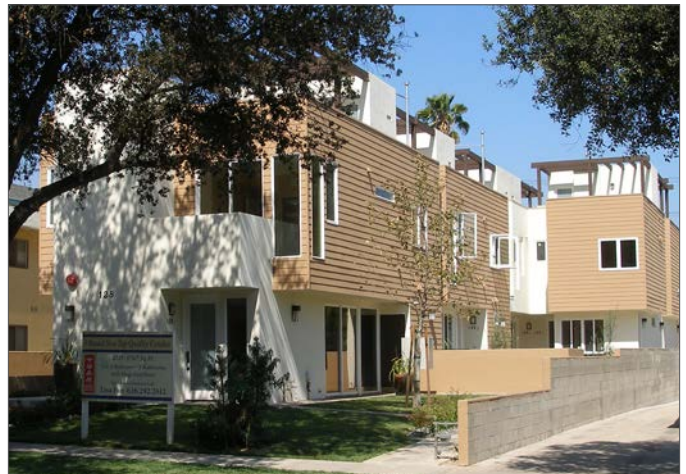
Trellises covered rooftop decks.
