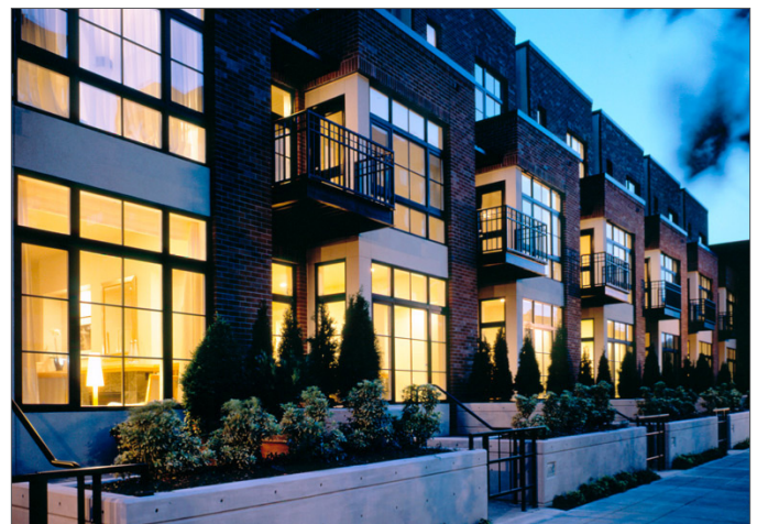
A multi-family building with two-story bay windows. The roof of the bay window is a balcony for the third floor space.
