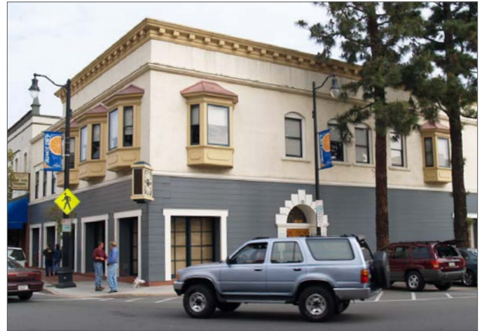
A mixed-use building with second-floor bay windows.
