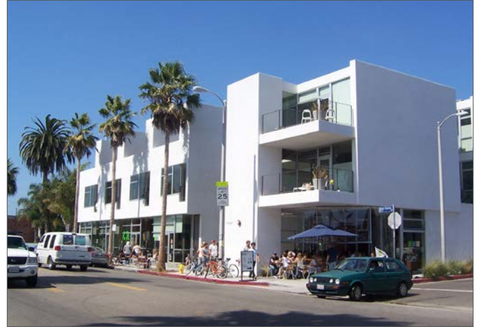
The massing of this mixed-use building is broken up by projecting corner balconies and chimney volumes that extend from the second floor residential units below.
