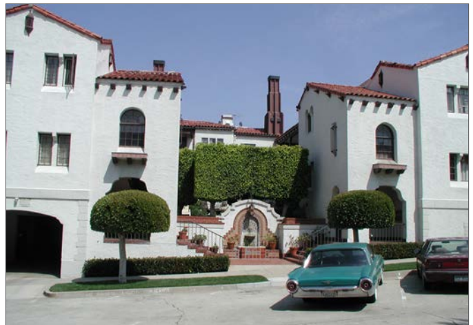
Example of an uncovered passage.
