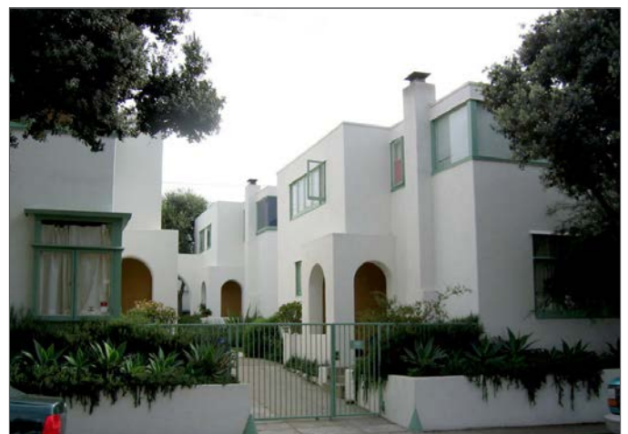
Building masses, entrance porticos, chimneys, and corner windows project from the main mass of this multi-family building.
