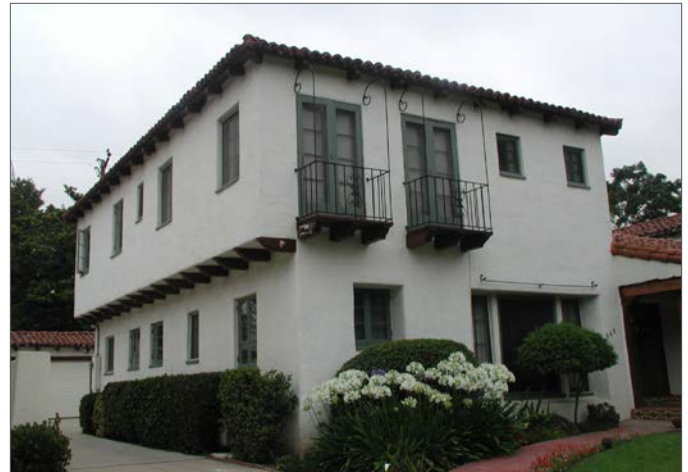
This building employs a couple of architectural elements to help break up the massing, including second-floor cantilevered rooms and street-facing, second-floor balconies.
