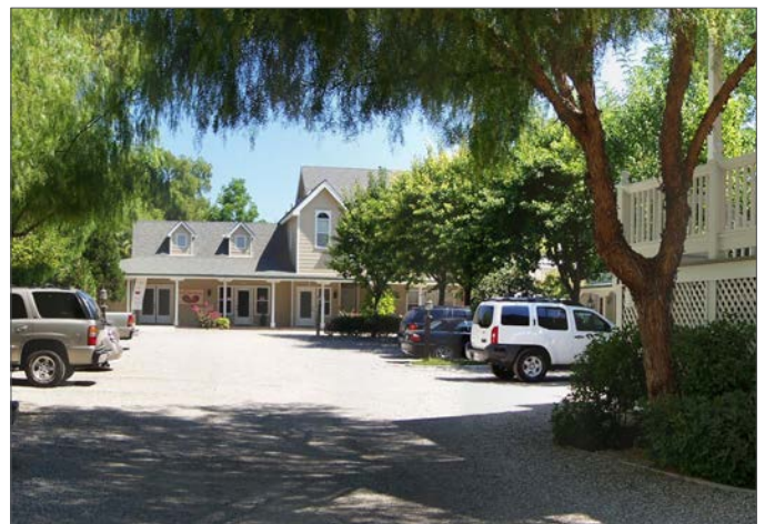
A parking lot paved with gravel and informal planting facilitates water recharging.
