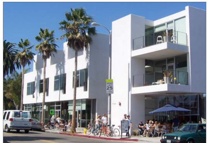
This contemporary building provides corner balconies to modulate the corner of the building and shade the shopfront below.
