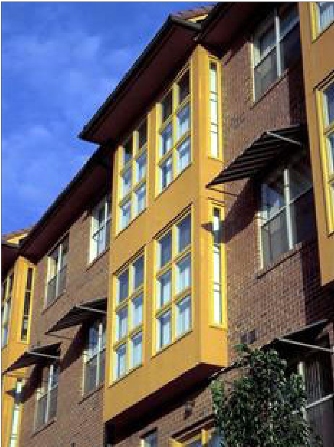
Example of a two-story bay window.
