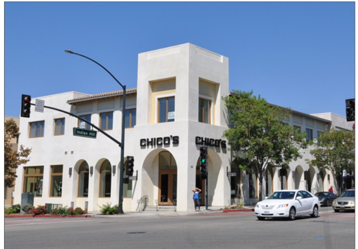
A combination of a prominent corner tower and building masses with parapets and pitched roofs reduced the apparent size of this building.
