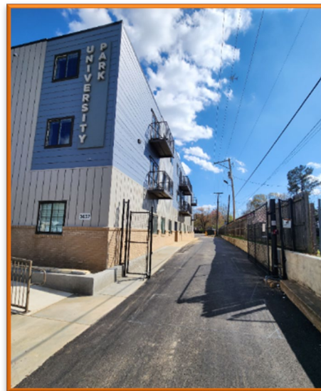
Security Gate Access
