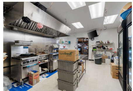
KITCHEN LINE AND HOOD
