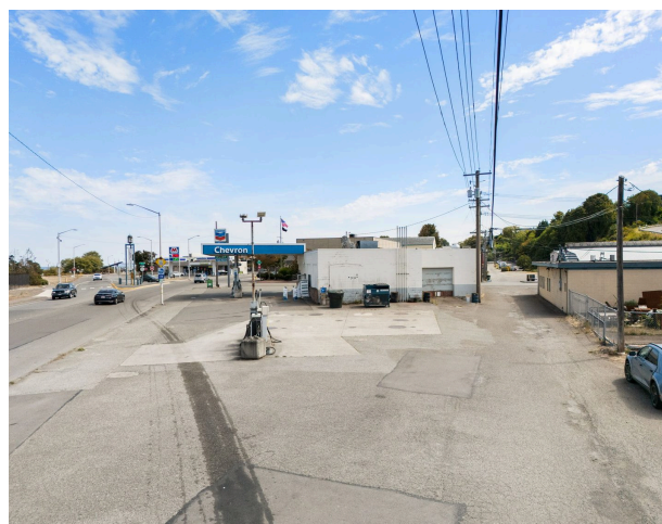
COMMERCIAL FUELING ISLAND IN THE REAR YARD, CURRENTLY OFFLINE
