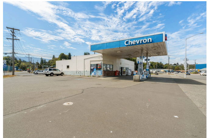
PAVED YARD AND SITE DEPTH
