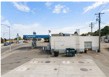
REAR YARD AND TRUCK ISLAND
