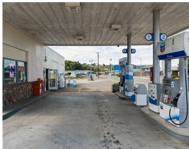
FOUR FUEL POSITIONS BENEATH THE CANOPY
