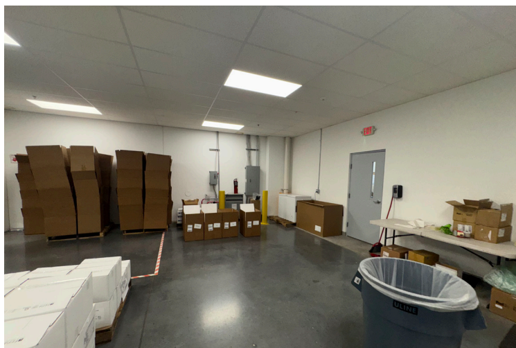
Temperature Controlled Air Condition Room
