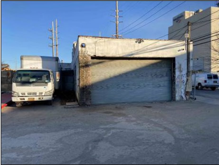
View of Improvements on Subject Lot 13 (Facing North)
