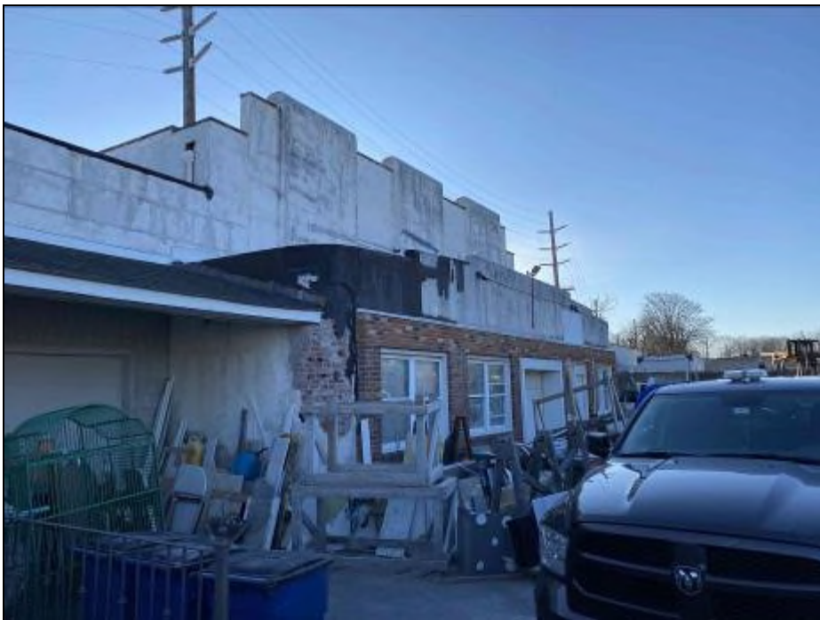
View of Rear of Improvements on Subject Lot 13 (Facing South)
