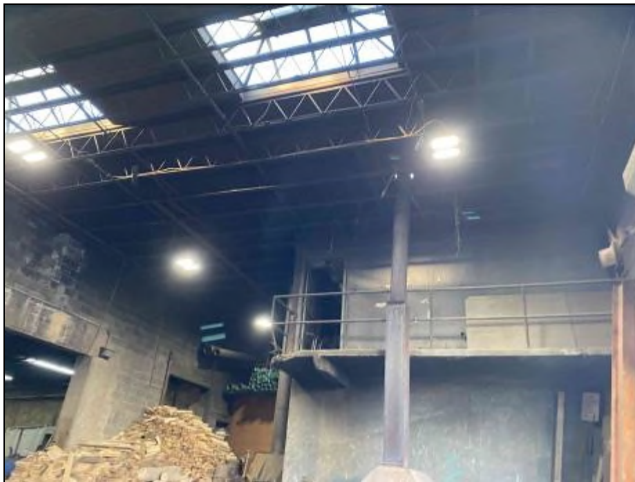
Interior View of Subject Property Mezzanine Improvements on Lot 11 (Industrial)
