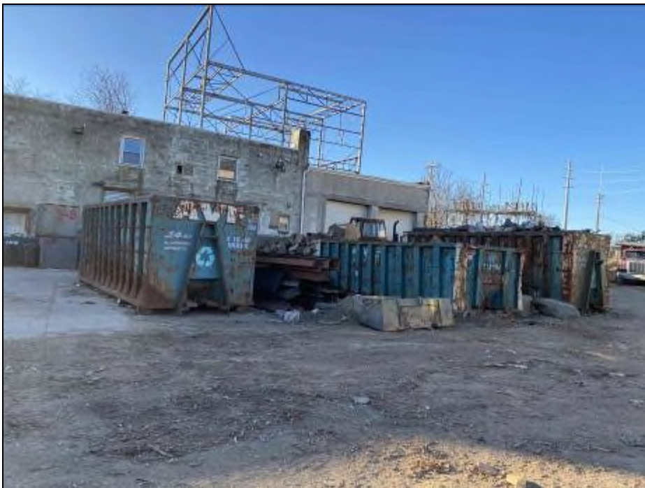
Exterior View of Subject Property Improvements on Lot 11
