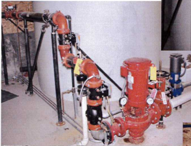
Water and Pump House: 15,000 gallons Fire Suppression System, Redundant Pumps Computerized controls.
