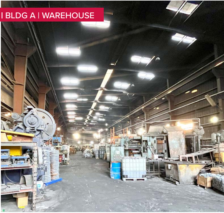
I BLDG A | WAREHOUSE CRANES
