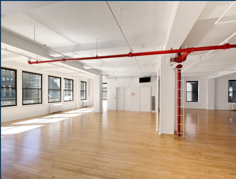
11th Floor - Existing Conditions
