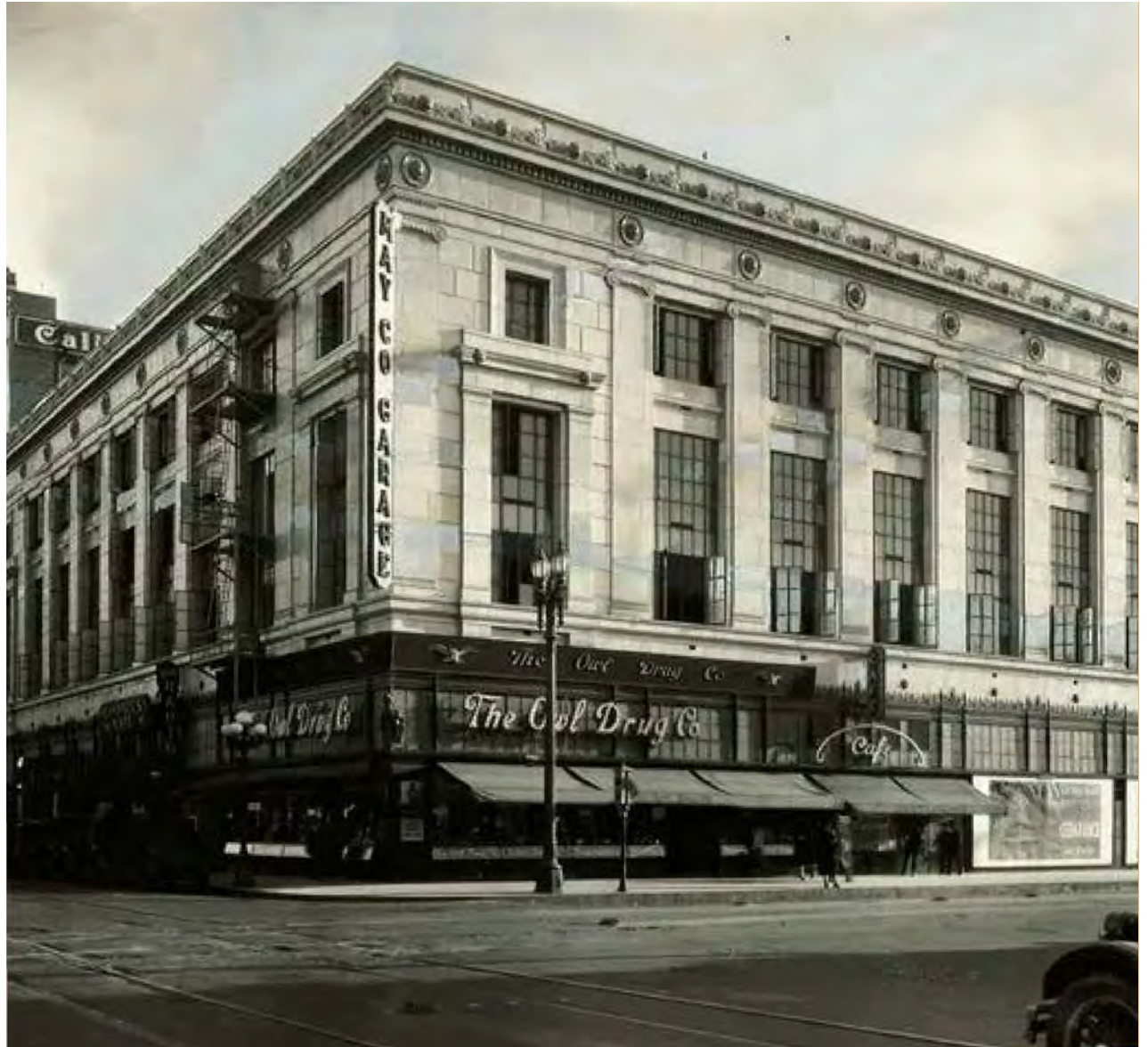
The Property upon opening as the May Company Garage in 1926.
