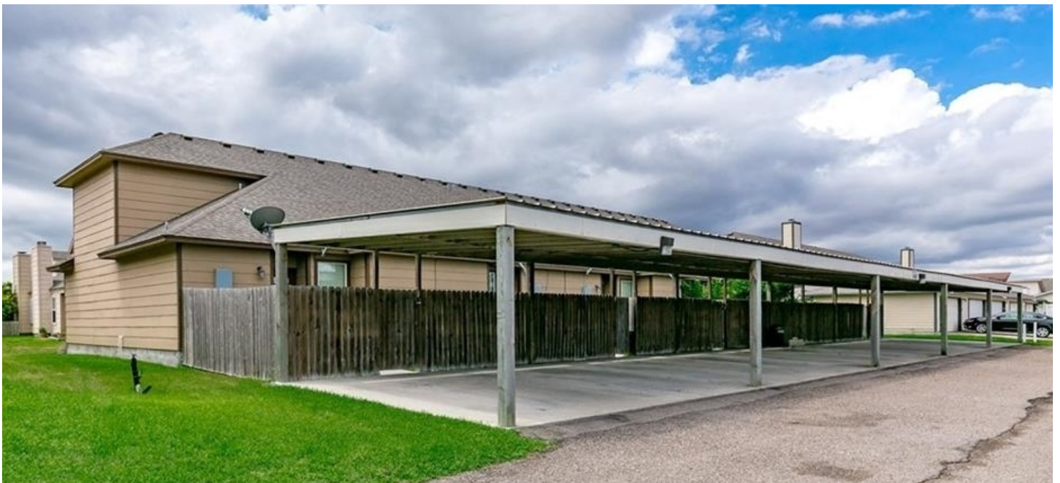
Each unit features covered carport parking, providing tenants with sheltered convenience and peace of mind.
