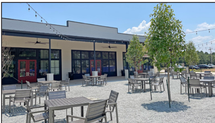
Windrush Village Phase 2 Building 1
