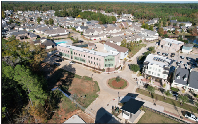
Town Center Roundabout
