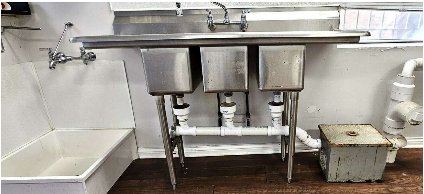
Triple Basin, Mop Sink and Grease Trap
