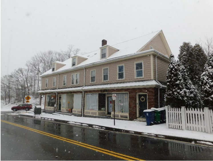
Front View of the Building
