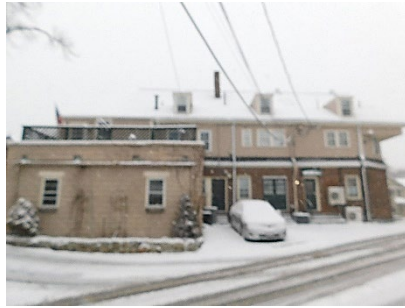
2. Rear of Building
