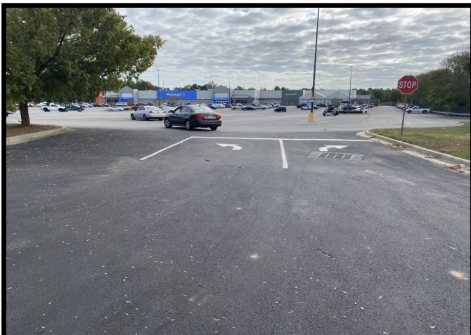
Ingress/Egress 2 out of parking lot
