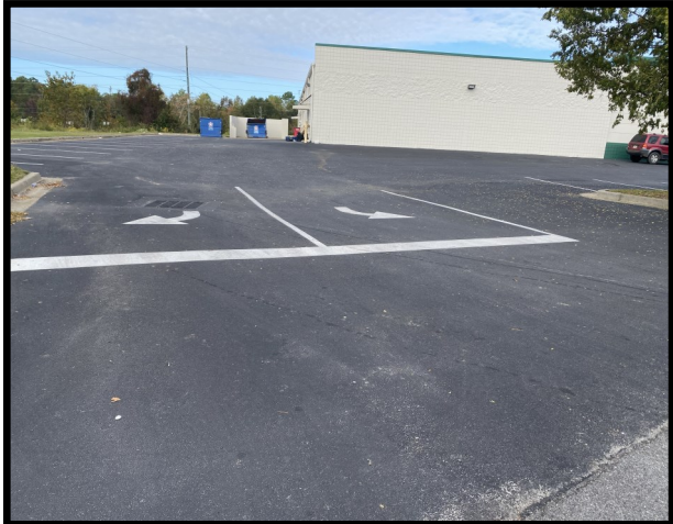
Ingress/Egress 2 into parking lot
