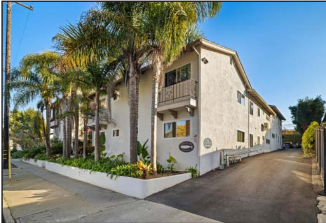
Front Exterior Showing Driveway With Parking Privately in Back
