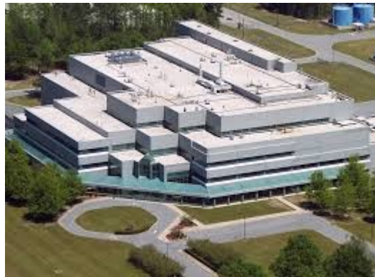
Large Industrial Facilities
