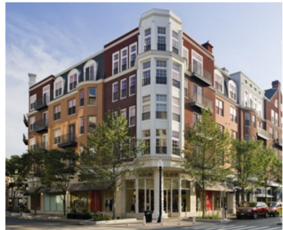
Mixed-Use Activity Center, Blue Back Square, West Hartford, CT (Image source: Turner, http://www.turnerconstruction.com/experience/project/19D/blue-back-square-mixed-use-development )
