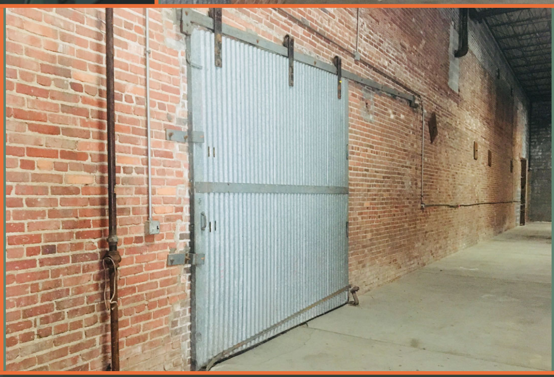
West Shared Wall
