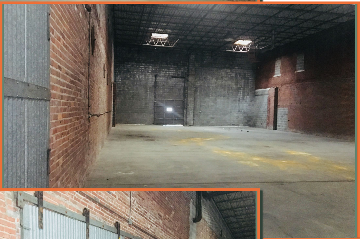
Warehouse Looking North
