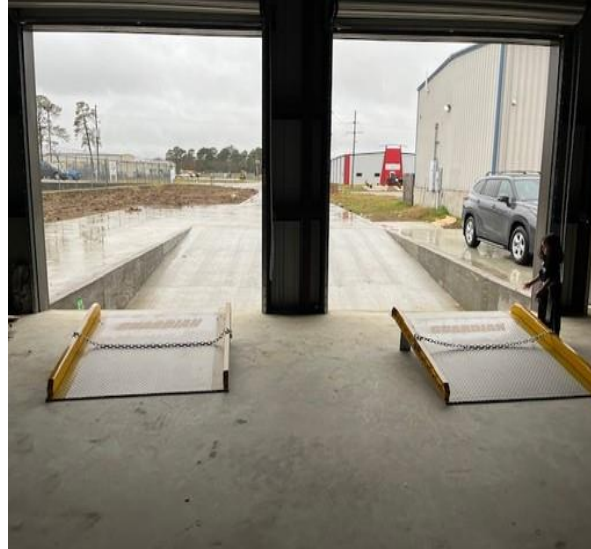
2 Truck Wells • Dock Levelers • 10'x10' Doors
