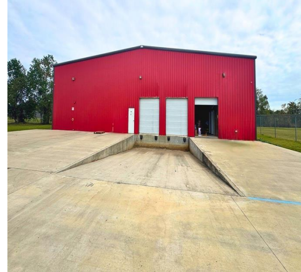
2022 Build • Concrete Apron • Expansion Land
