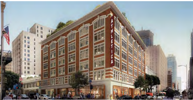
712 OLIVE Building Conversion to Creative Office (1 Block Away)
