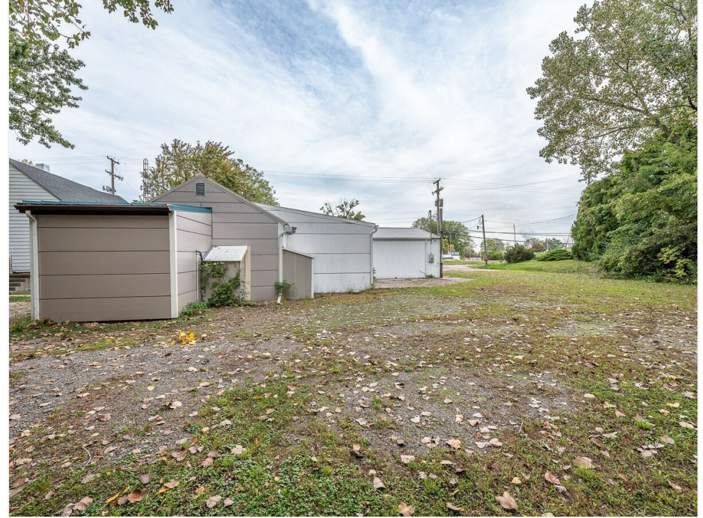
Back of Building
