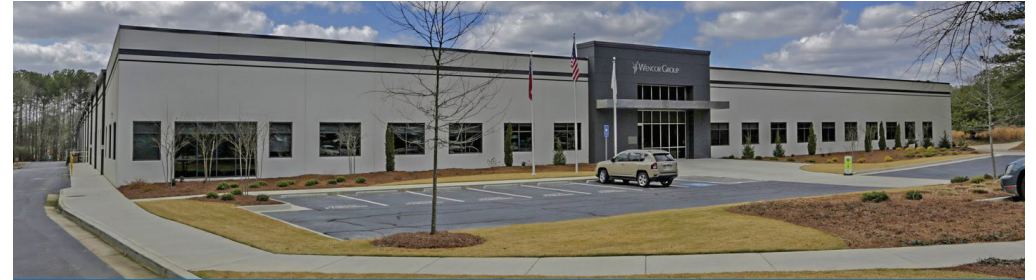
Government Contractor Facility | Peachtree City, GA (±163,000 SF)
