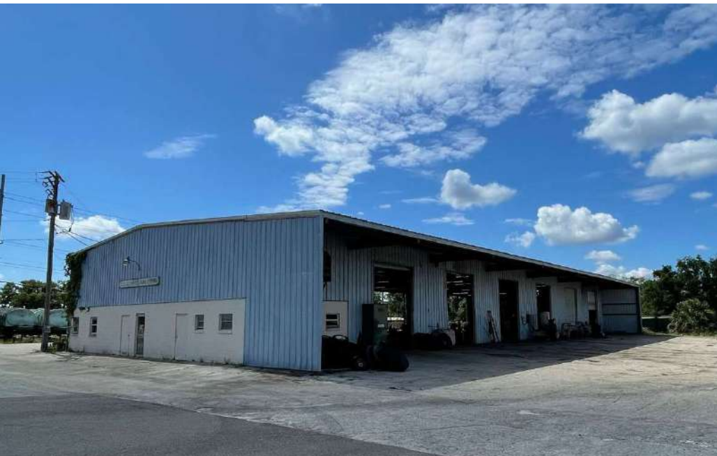
Service & Repairs Building
