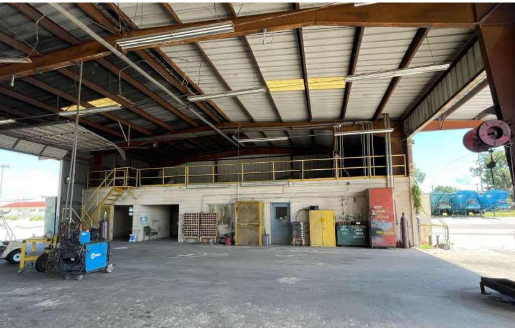
Service & Repairs Building
