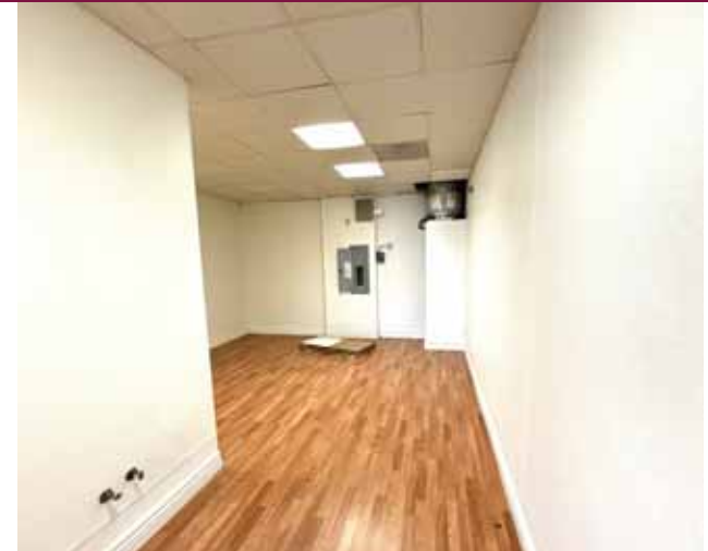
2652-E Interior - Plumbing Stub Outs
