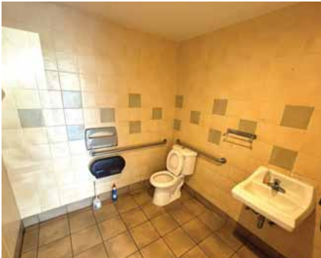
2652-E Interior - ADA Restroom Upgraded Tile Floor/Walls
