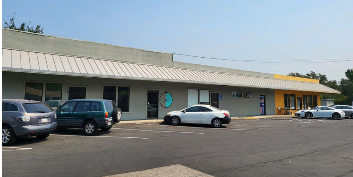
SIDE OF BUILDING
