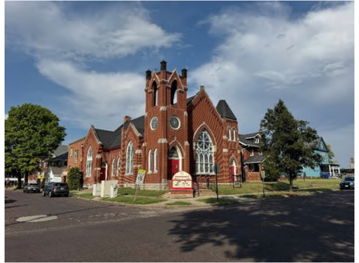
FRONT VIEW OF MAIN BUILDING
