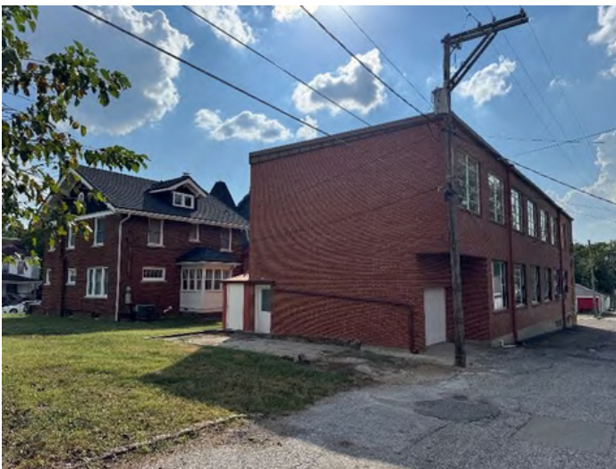
REAR VIEW OF MAIN BUILDING AND PARSONAGE
