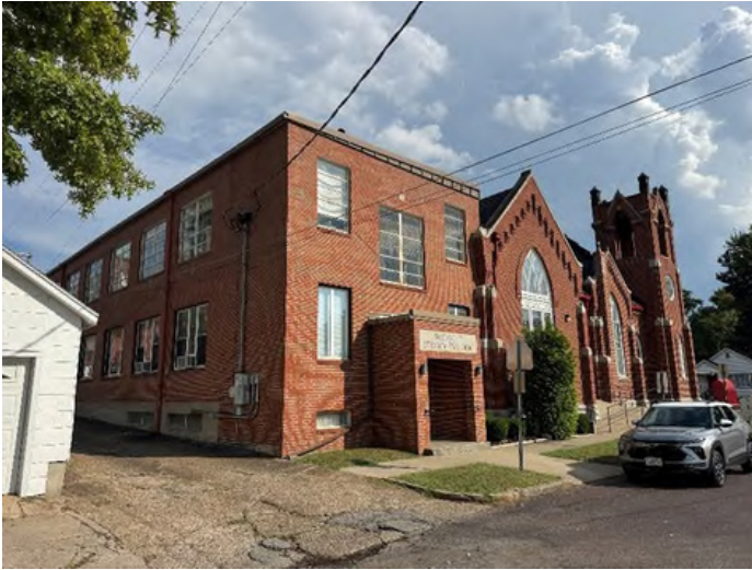
FRONT VIEW OF MAIN BUILDING
