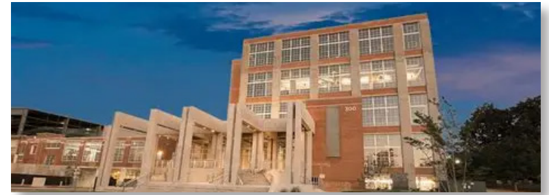
The Lowenstein Building
