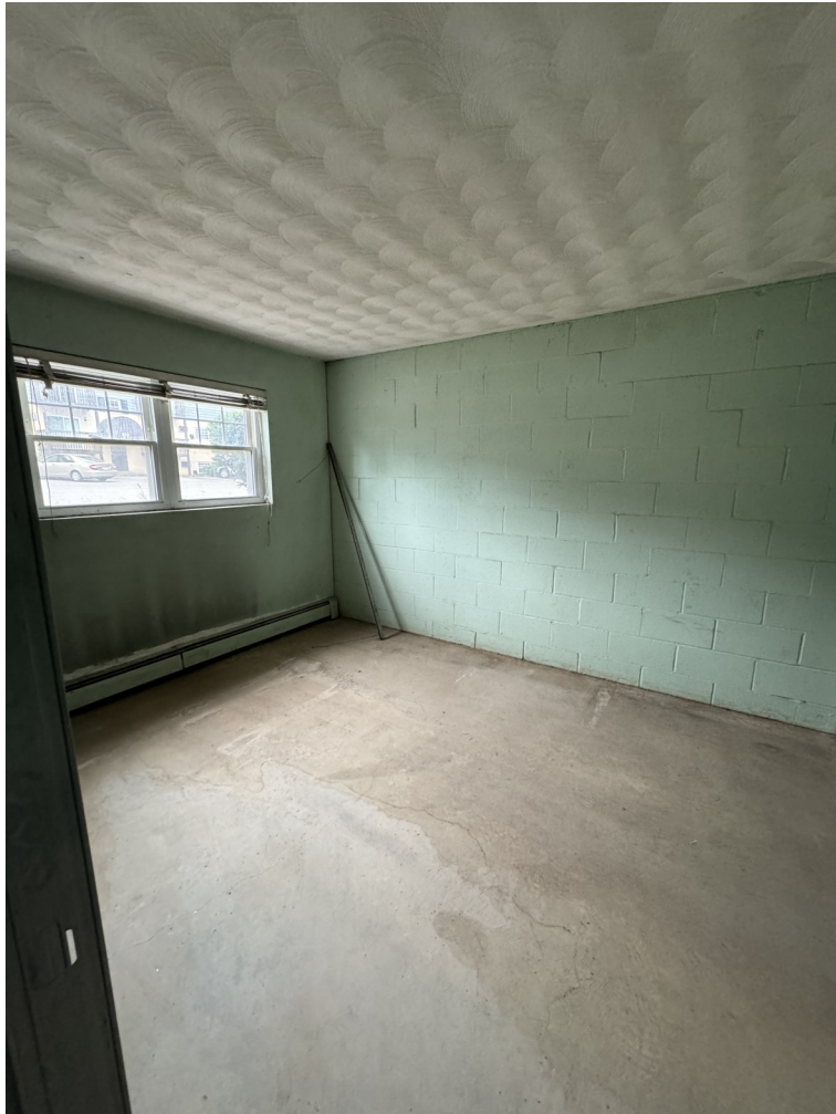
View From Hallway into the Bedroom
