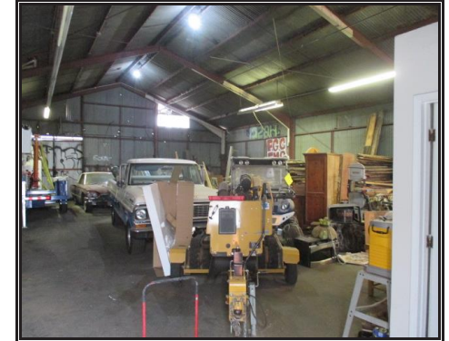
Metal Building – Interior.
