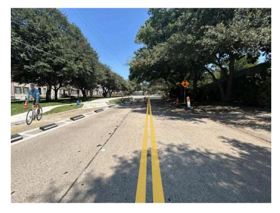
Work on the Beltway Trail Project continues to move forward. Since construction began in February, crews have completed concrete walking trails, off-street bike lanes, traffic calming features, sidewalk connections, and light pole installation. Upcoming work includes planting, roadway striping, and bike lane protectors.
