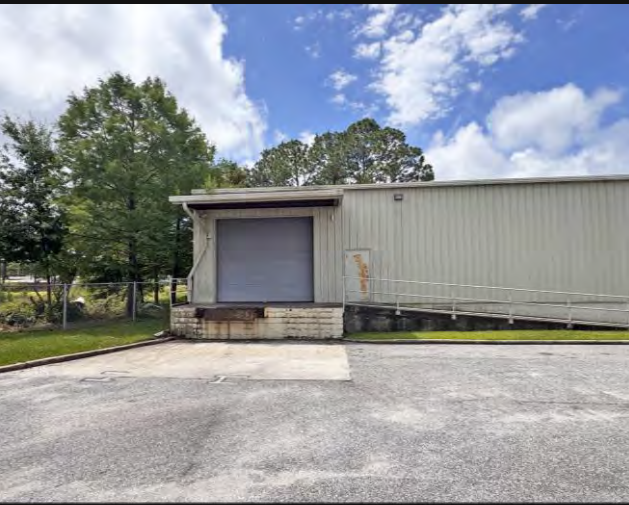
WAREHOUSE — LOADING DOCK
