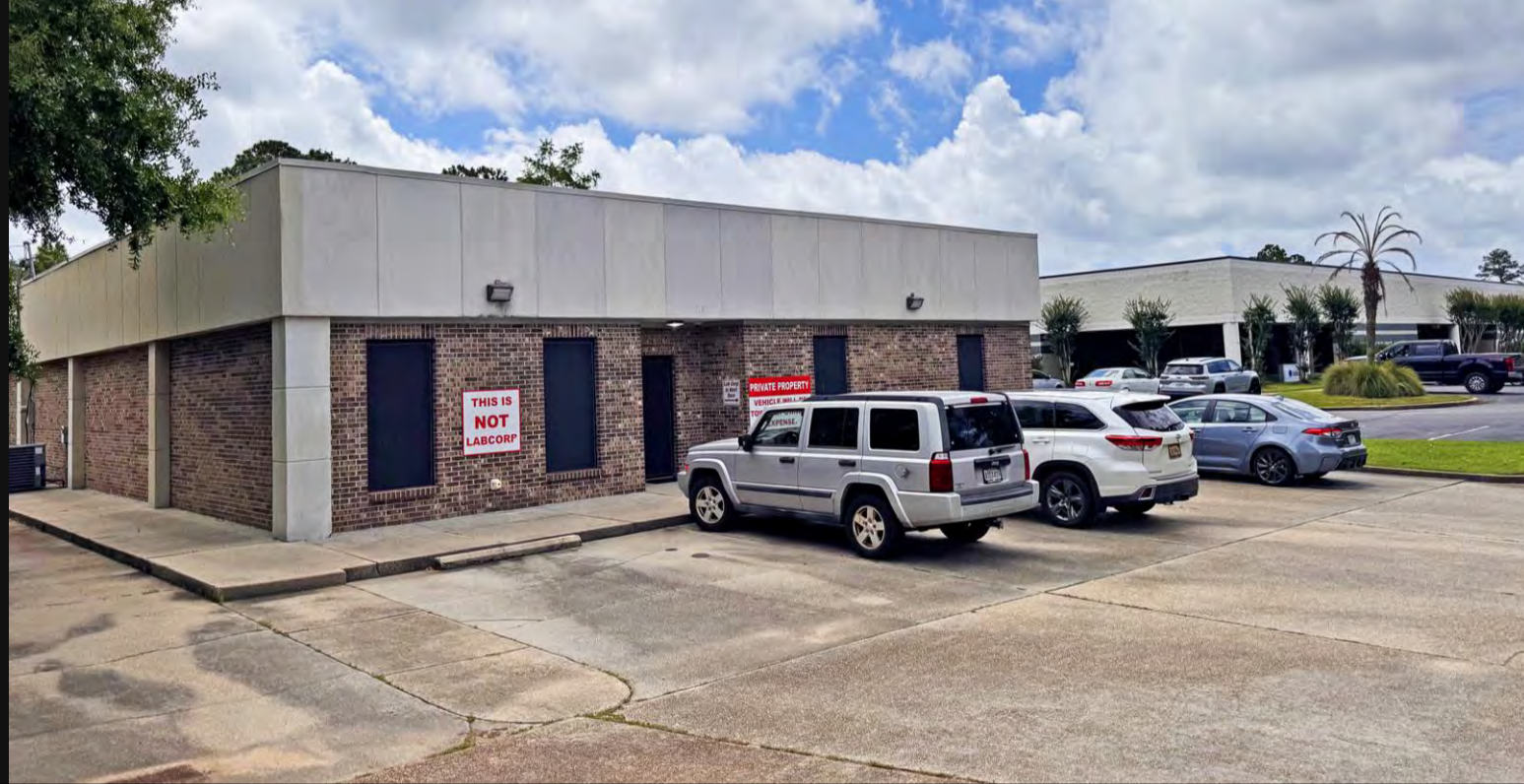
EXTERIOR — 1181 MONTLIMAR DRIVE
