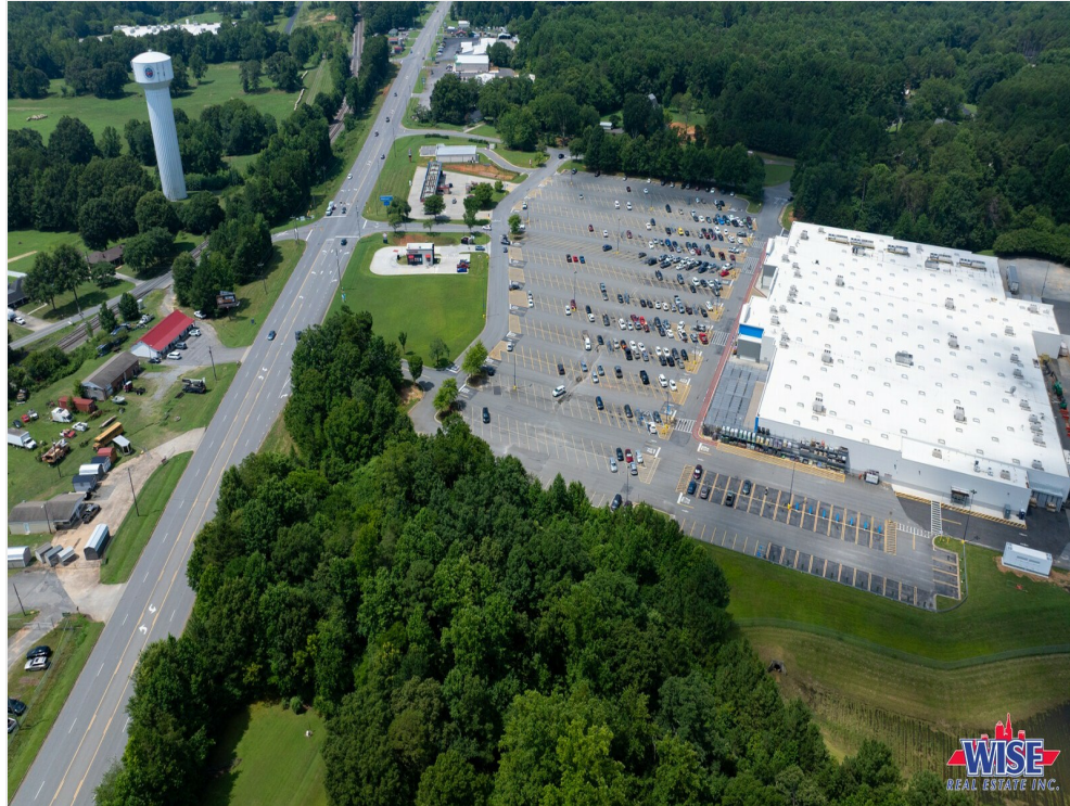
Aerial Facing West
