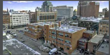
Back of Building
