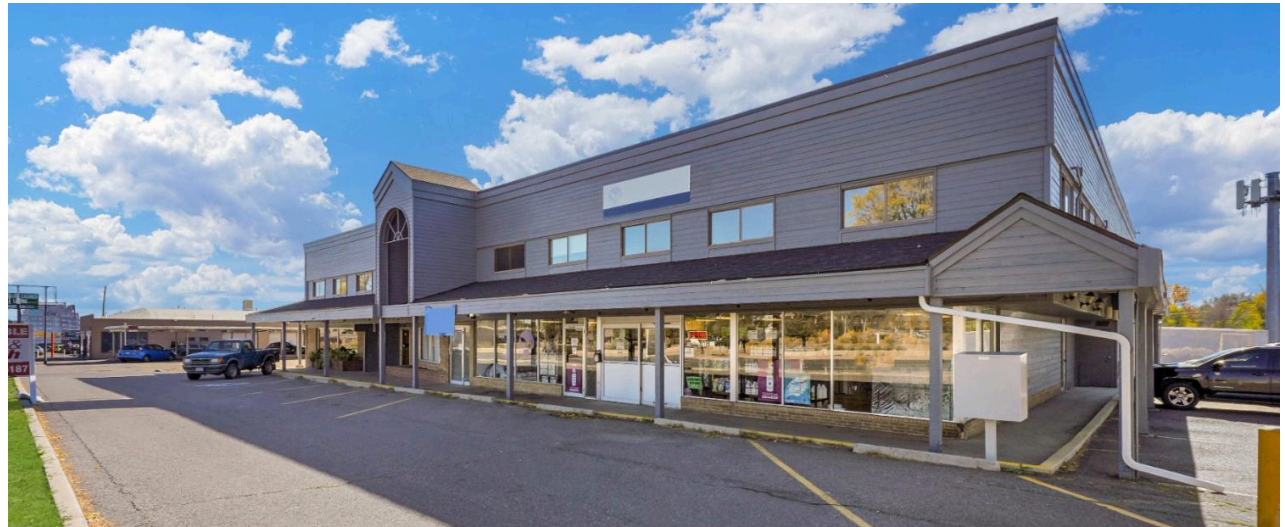
8646 W COLFAX AVE — GROUND-FLOOR STOREFRONT RUN AND COVERED WALKWAY
