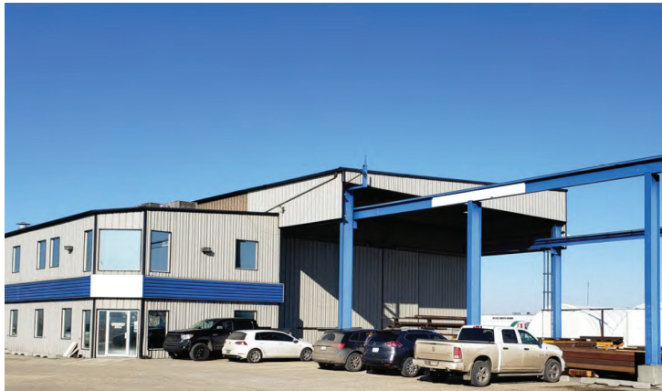
Outdoor crane way
