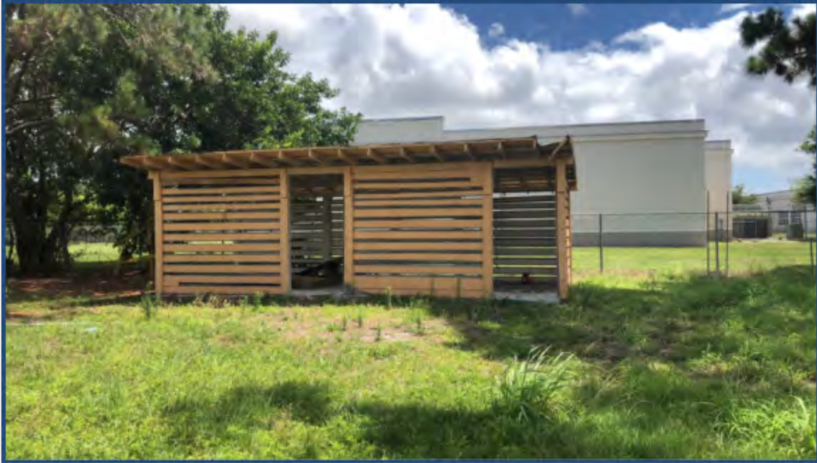
Photograph 11: Storage Shed in Southeastern Corner of Subject Property
