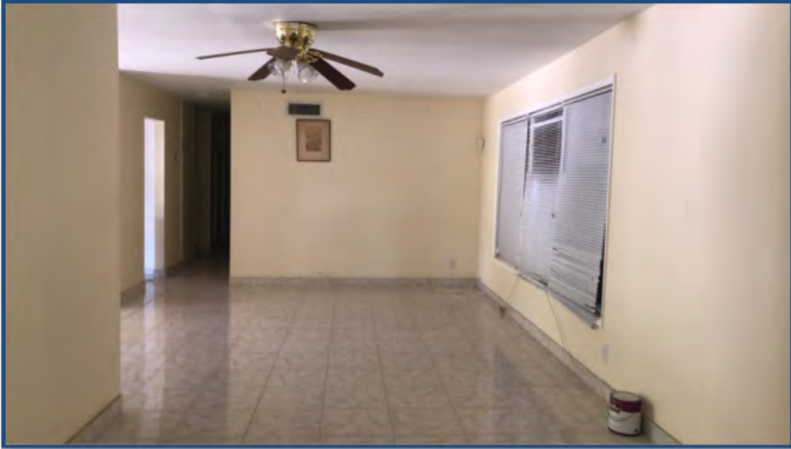
Photograph 23: Interior Living Space
