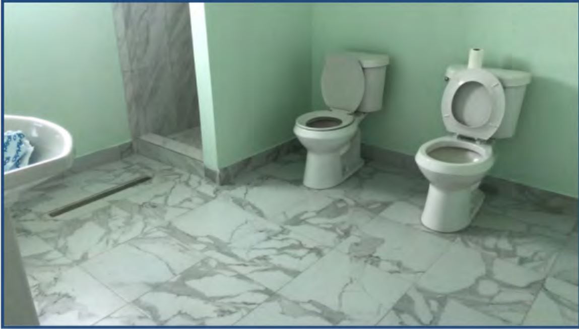
Photograph 7: First Lavatory with Floor Drain and Shower Drain
