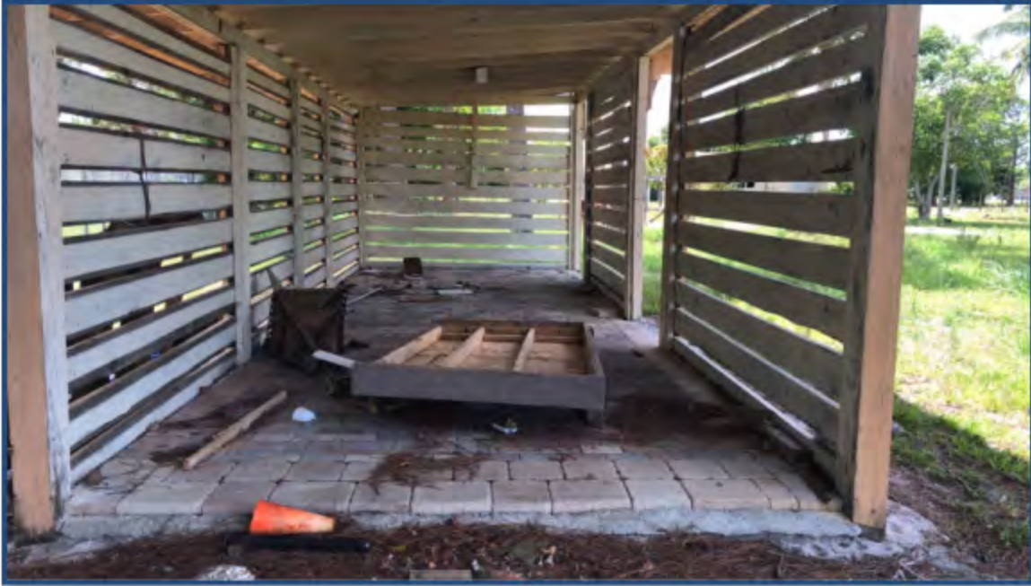
Photograph 13: Interior of Storage Shed
