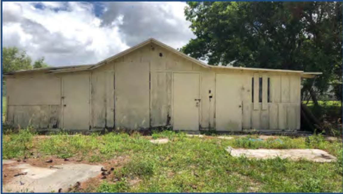
Photograph 15: Second Storage Shed in Southeastern Corner of Subject Property
