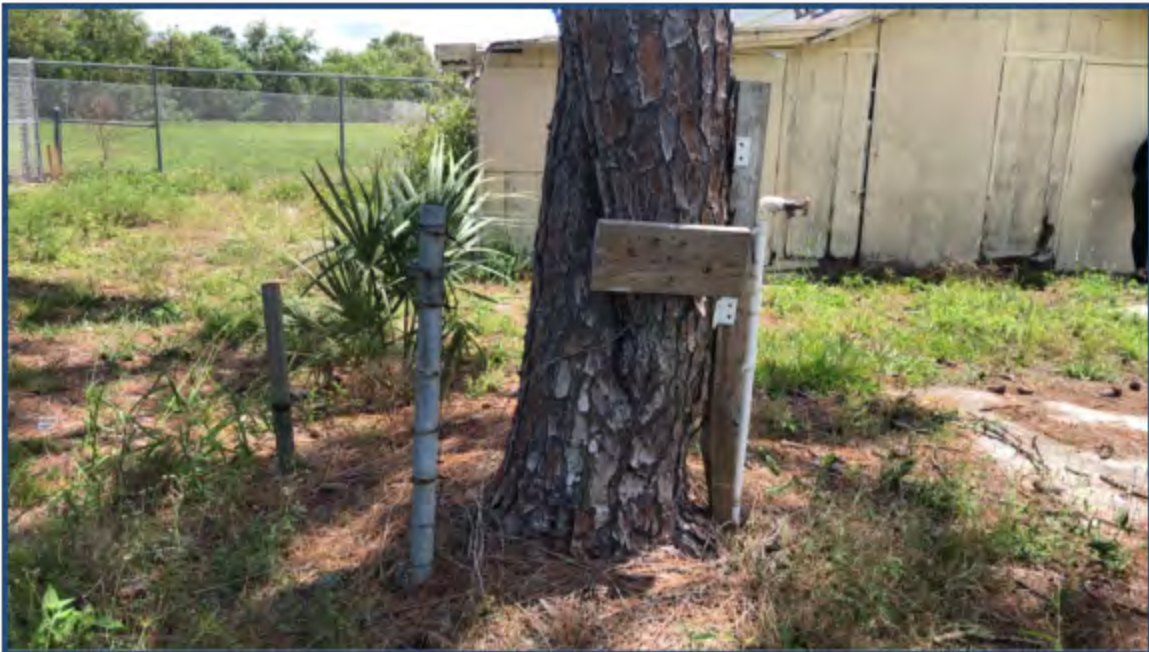
Photograph 18: Irrigation Pipe in SW Corner of Subject Property
