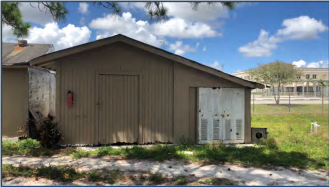
Photograph 29: Storage Shed adjacent North of Vacant Single Family Home
