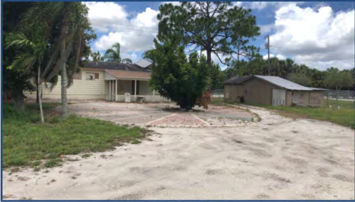
Photograph 19: Vacant single-family Home and Two Storage Sheds in Northwestern Corner of Subject Property
