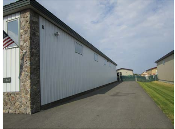
Photo #2 View looking west at the north side of the Site building.
