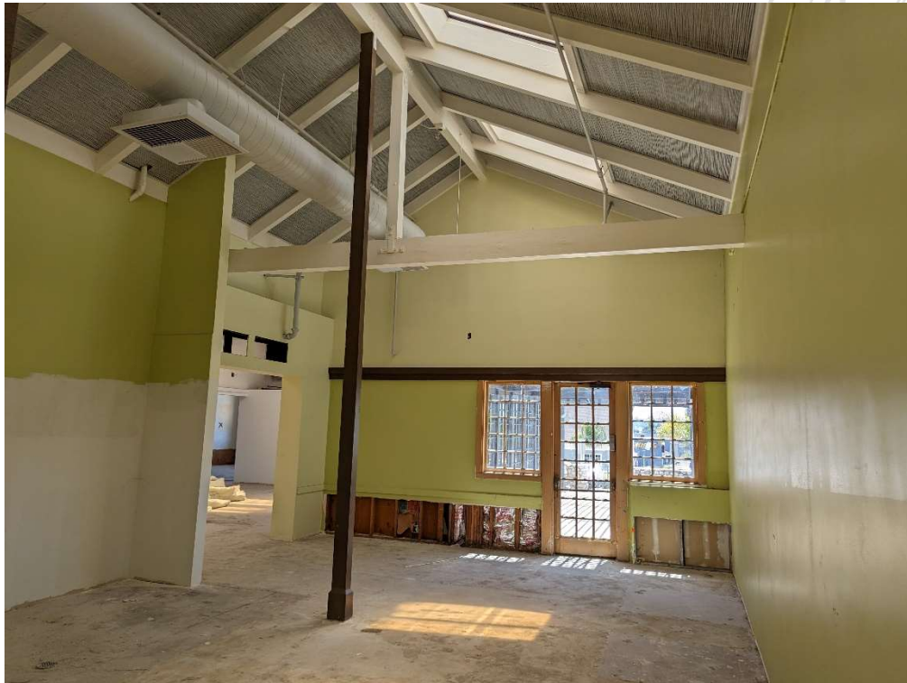
Vaulted Ceilings and Skylights
