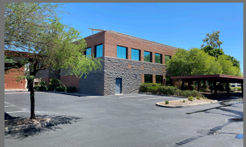
Parking Lot Resealed
