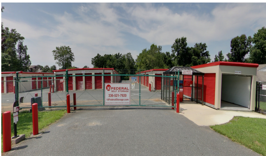
Gated and well secured
