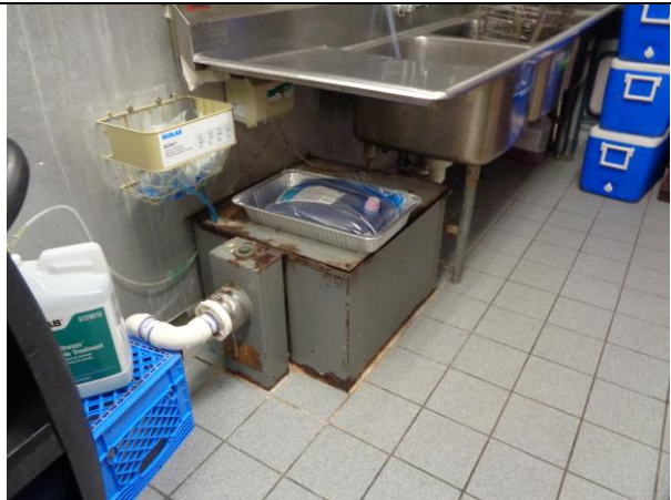
(12) View of Kitchen Grease Trap
