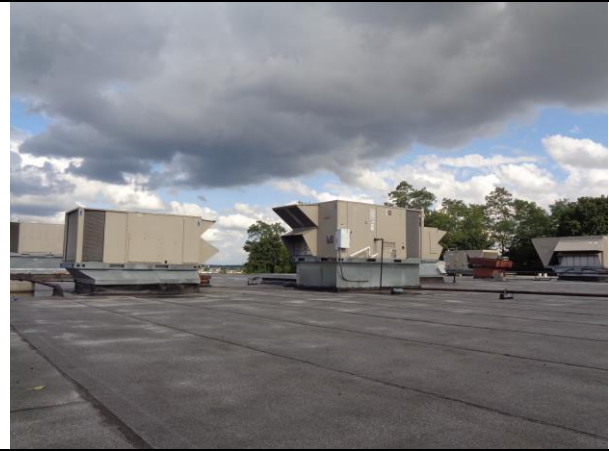
(22) View of Roof
