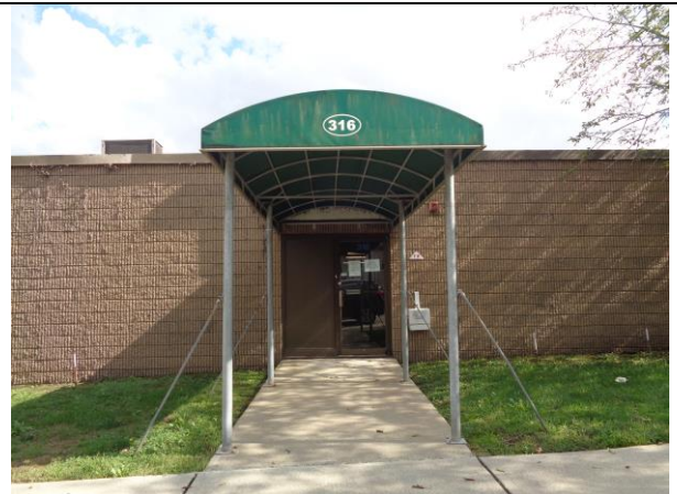
(18) View of Entrance of Vacant Offices
