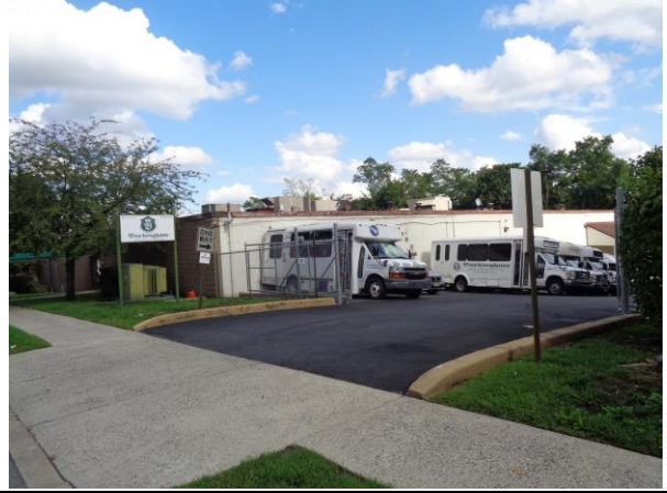
(2) Easterly view of the subject property
