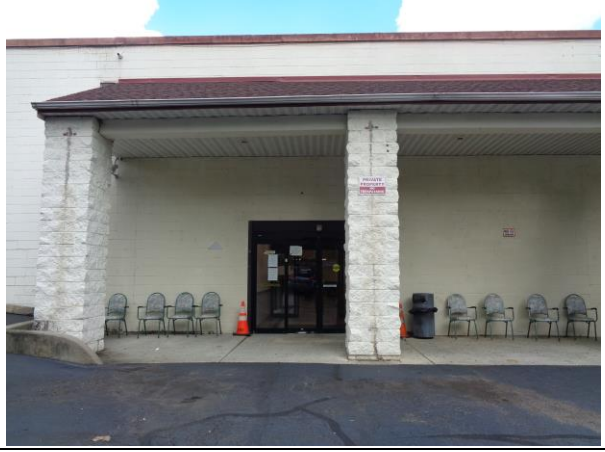
(8) View of Entrance of Daycare Center
