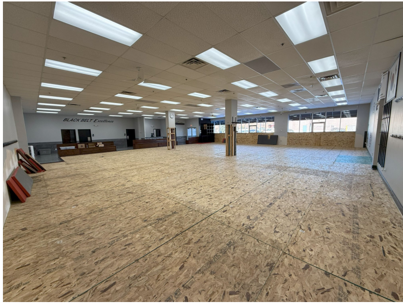
Main Open Area — High Ceilings
